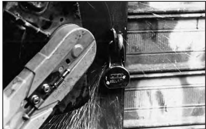
(Below) Cutting the hasp from the channel rail. Do not cut the pin! Pull out the lock and pin.
