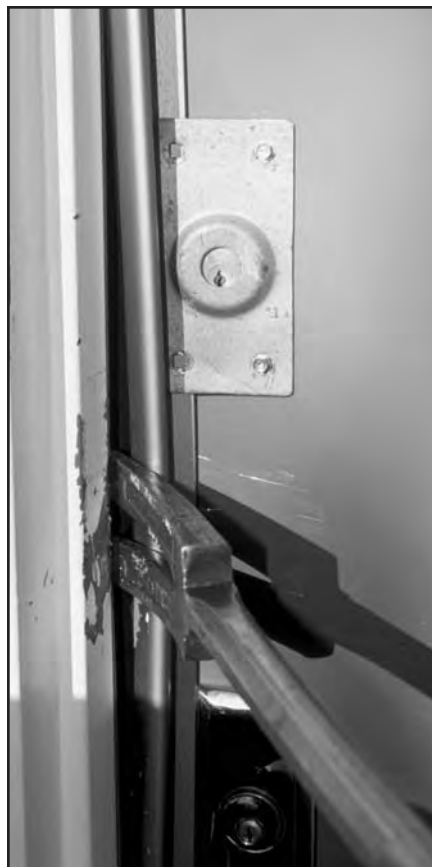
Figure #10--The technique is modified by driving the fork of the Halligan between the shield and the door frame.
