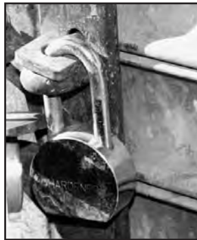
(Above) Case-hardened padlock secures a removable pin to the guide rail.
