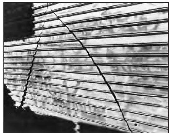
(Right) The top of the second cut is left unfinished until both sides are cut. Then, join the cuts. This allows the gate to stay in place during operations.
